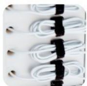
Individual velcro cable fasteners secure cables in place
