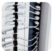
USB cables are connected in the side locked compartment
